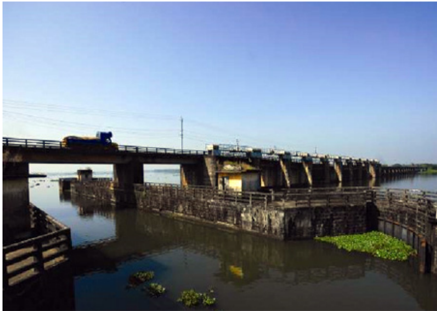
Thannermukkom - Salt water barrier
